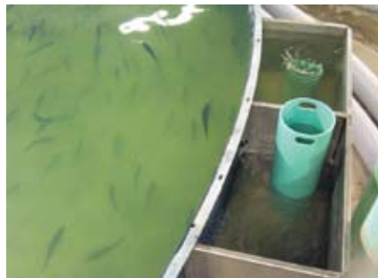
Left: Sidewall Drain and Mortality Box. Right: Pneumatic Mortality Drain.
